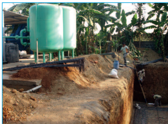
Digging the tanks for recycled water.
